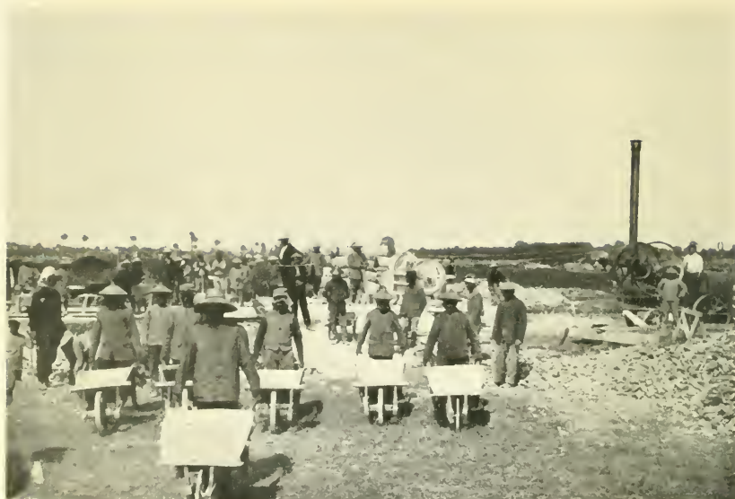
Tank Factory, Neuvy Pailloux, France. ( p. 220)
